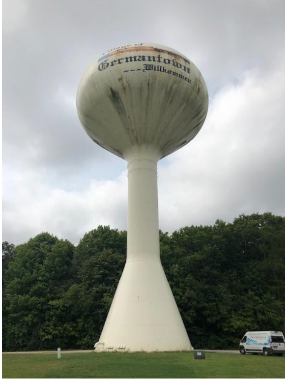
Germantown Water Utility – WIDNR 5 Year ROV Water Tank Inspection – 1 MG Sphere - 2020
