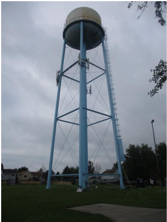
Kenosha Water Utility – WIDNR 5 Year Drain & Clean Out Inspection – 100k Legged - 2020
