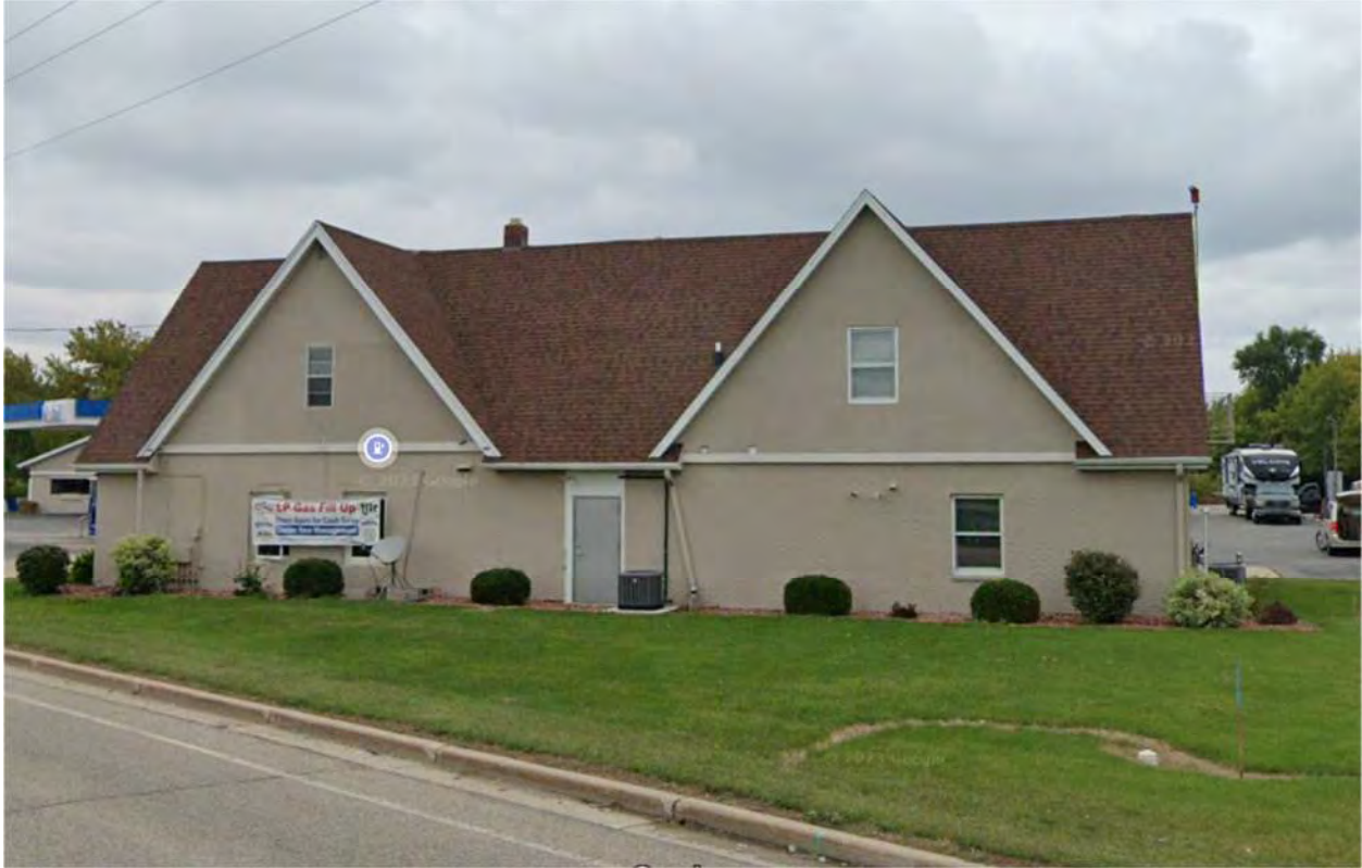
EXISTING SOUTH FAÇADE – NORTHWESTERN AVE.
