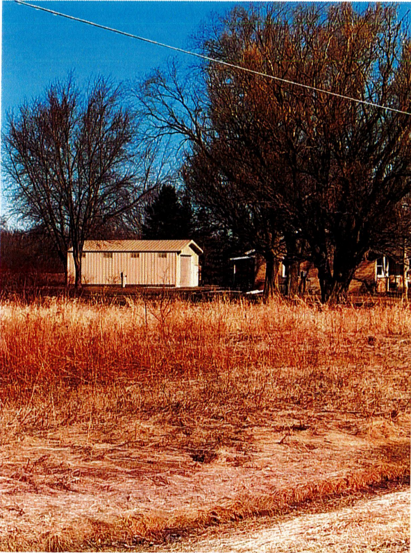
Existing Pole Barn on Bay Filly Lane
