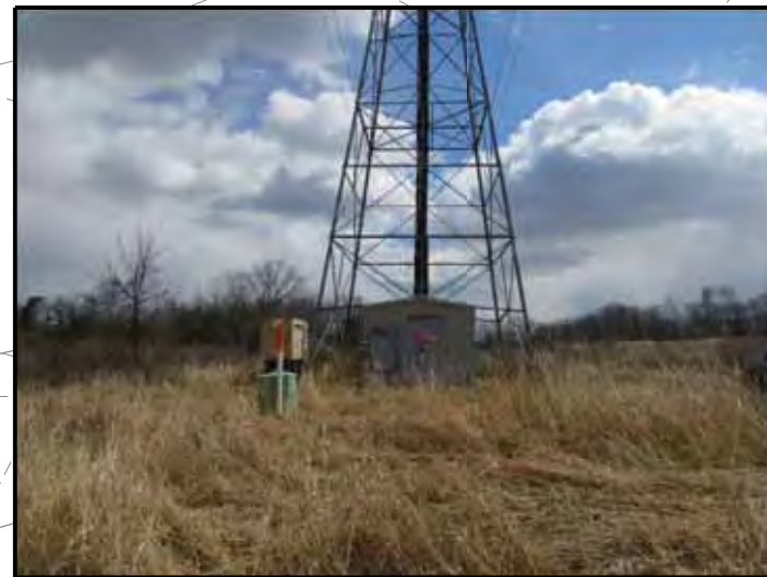
SITE OVERVIEW (LOOKING EAST)
