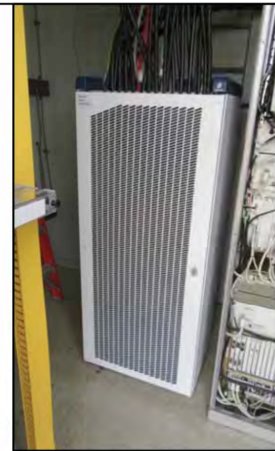
EXISTING LTE EQUIPMENT CABINET
