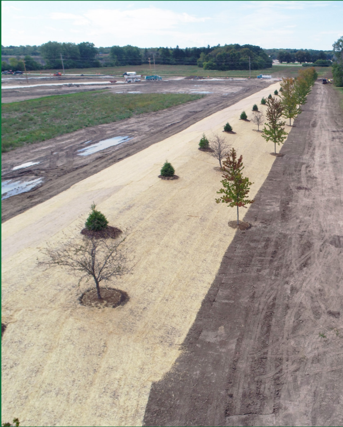
New headlight screening berm - looking west.
